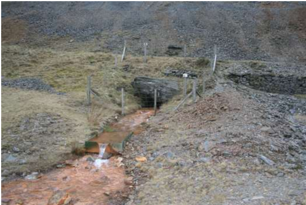
Water draining from Pugh's Level (iron oxide causing the red colouration)
