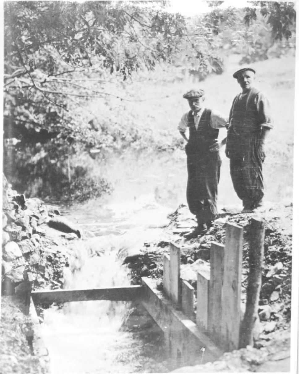
Leat Wall 'swallow' "B" showing water pouring down 'swallow' before filling.
